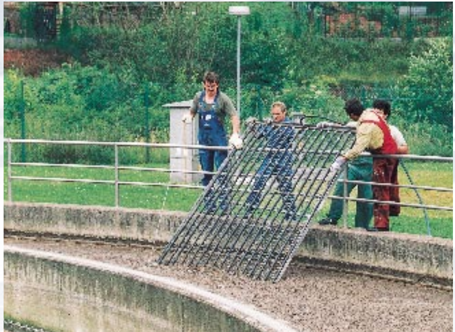
Installing an oxygenation mat in an activated sludge tank
