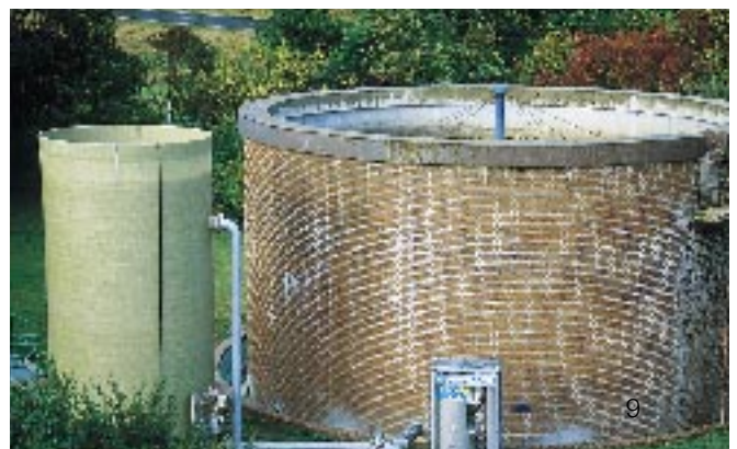
Prepurification of waste water before transfer to a trickling filter plant
