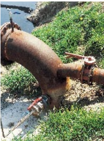
“Aerobic sealing” of waste water lagoons
